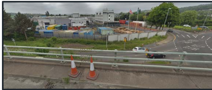
Figure 29: Outfall 9 Street View (Google)
