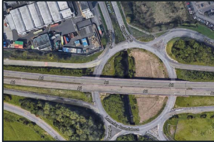
Figure 28: Outfall 9 Aerial View (Google)
