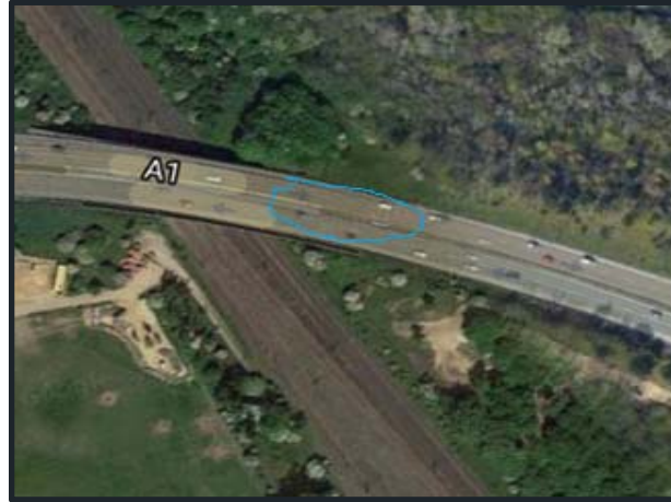
Figure 25: Outfall 8 Aerial View (Google)
