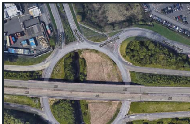
Figure 31: Outfall 11 Aerial View (Google)
