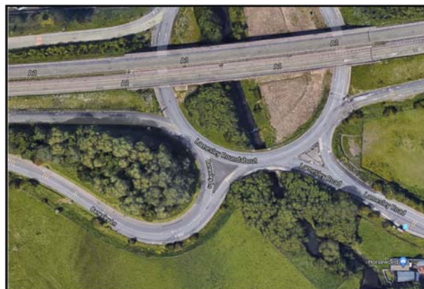
Figure 37: Outfall 13 Aerial View (Google)
