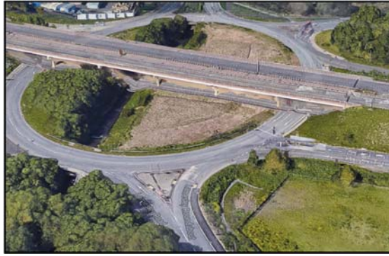
Figure 38: Outfall 13 Street View (Google)
