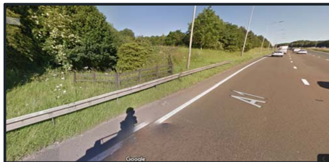
Figure 21: Outfall 7 Street View (Google)
