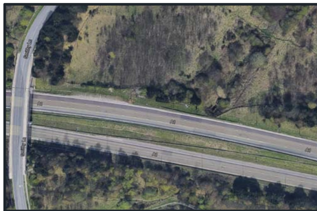
Figure 20: Outfall 7 Aerial View (Google)
