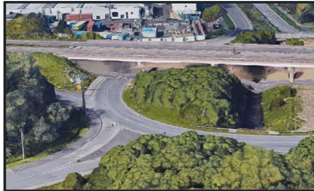
Figure 35: Outfall 12 Street View (Google)
