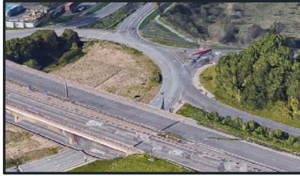
Figure 32: Outfall 11 Street View (Google)
